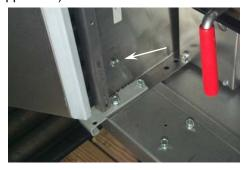
Figure 6. Cabinet connection locations inside cabinet sections (front shown).
